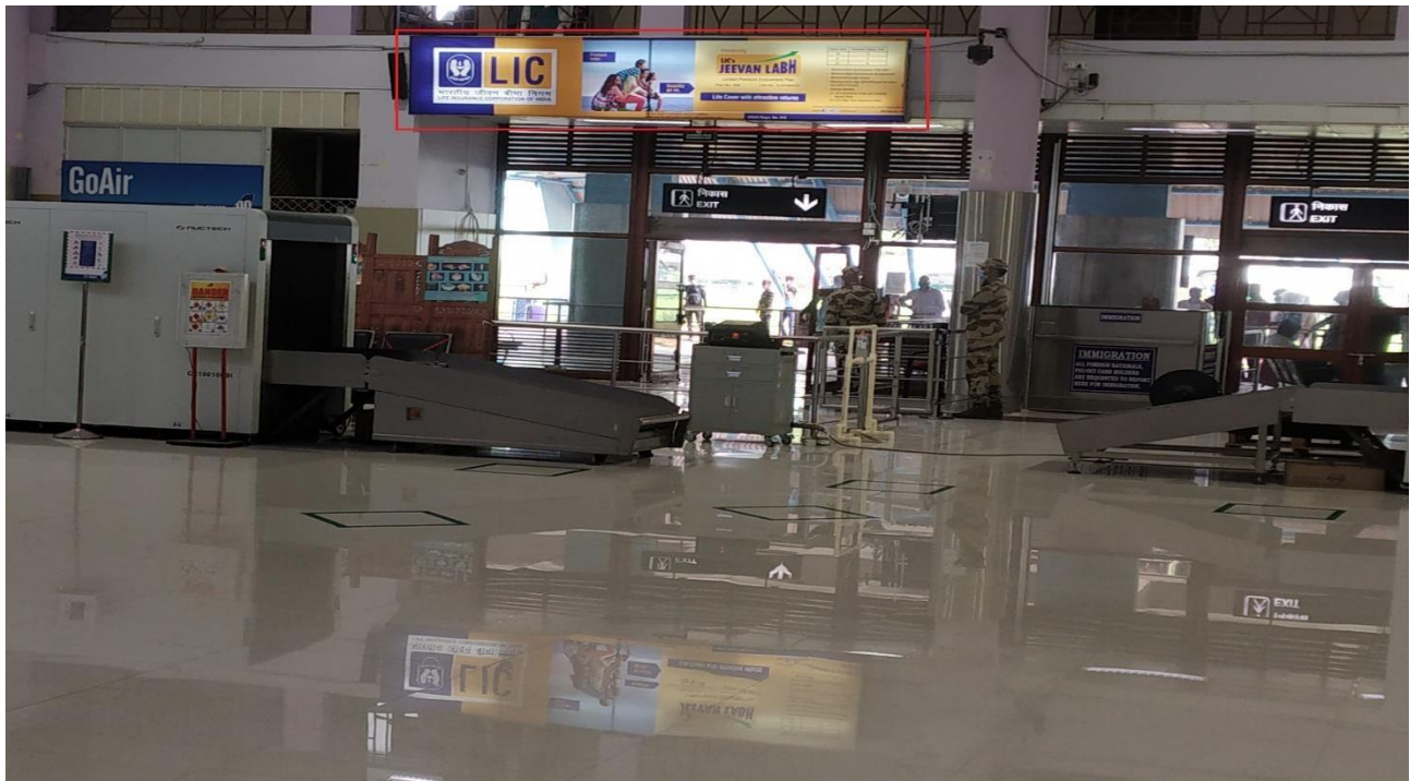
Slide No. 12 - Wall Portion in Arrival Hall Above Arrival Exit Gate towards Cityside (5m x1m) (53.82 sq. ft)
