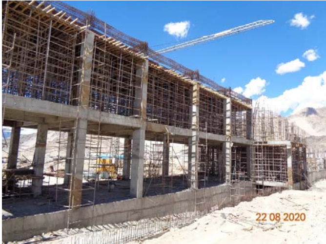
Construction of Utility Building in progress
