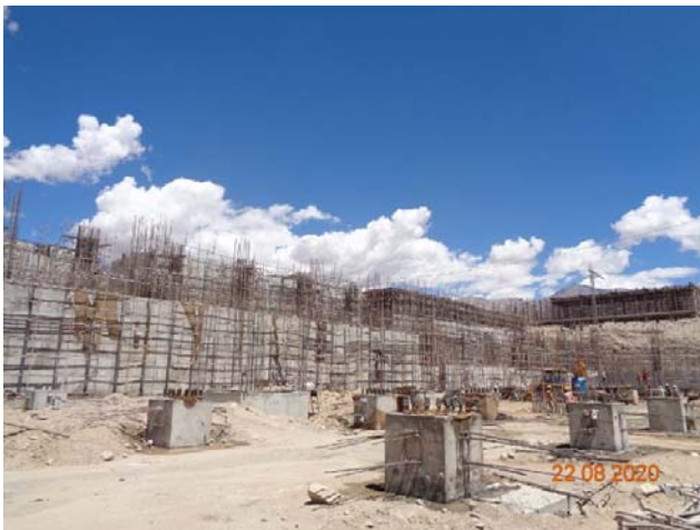
Construction of Terminal Building in progress
