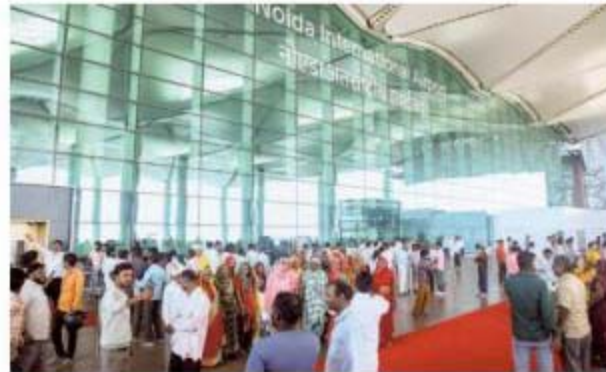
PUBLIC RESPONSE. People gather at the newly constructed Noida International Airport after its inauguration by Prime Minister Narendra Modi in Jewar, UP, on Saturday.
