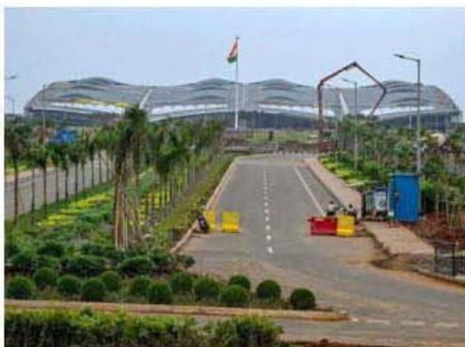
READY FOR BUSINESS. Bhogapuram international airport, near Visakhapatnam
