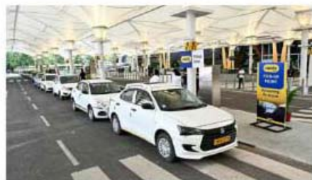
Some of the infrastructure projects at the Chennai airport were inordinately delayed before they were finally opened. A case in point was the cab pick-up point. FILE PHOTO
