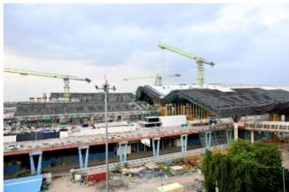
Frustrating wait: Passengers also ask why the deadline for the construction of the T3 Terminal has been extended many times. AAI officials say the facility will be ready in seven months. M. SURESH
