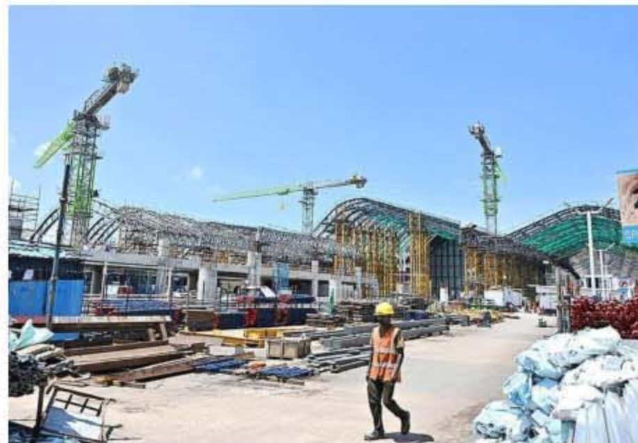
Work under way at the T3 International Terminal of the Chennai airport. B. VELANKANNI RAJ
