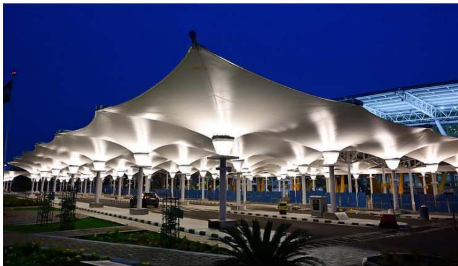
The second cab pick-up point is located inside the plaza opposite the T1 domestic terminal. B. VELANKANNI RAJ
