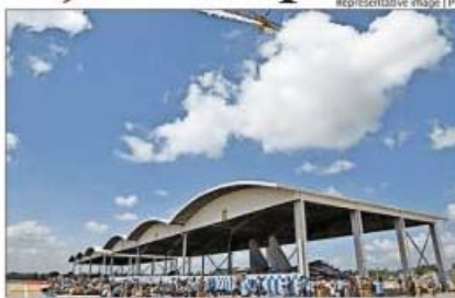
AWAITING NOD TO BEGIN WORK: The plan includes a passenger terminal, a link taxiway and aircraft parking bays
