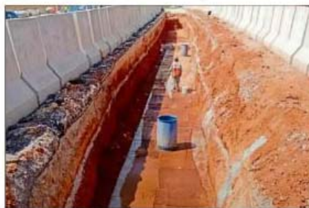
A view of works undertaken for the vehicle overpass at Sadahalli Junction on the airport road.
