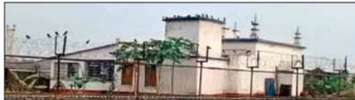
Bankra Mosque inside Netaji Subhas Chandra Bose International Airport
