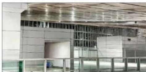
An area next to the lounge where the expansion is being planned
