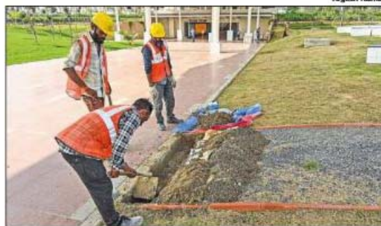
Work under way to ensure rainwater does not reach the walkway
