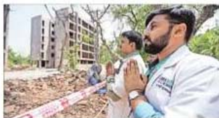
Outside the hostel buildings that were struck during the plane crash, in Ahmedabad on Friday. (AP/POD/ANSA)
