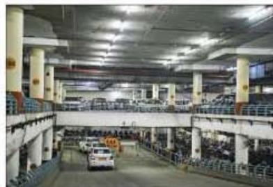
The airport car park, where painting and maintenance work is being carried out
