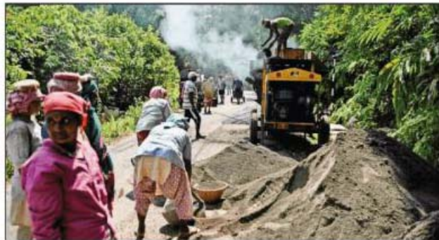
Construction workers in Great Nicobar Island on March 26
