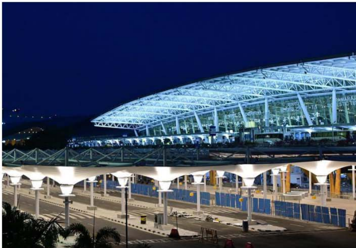
Rest area: The plaza, located opposite the T1 domestic terminal, contains walkways and seating spaces for air passengers and visitors. B. VELANKANNI RAJ
