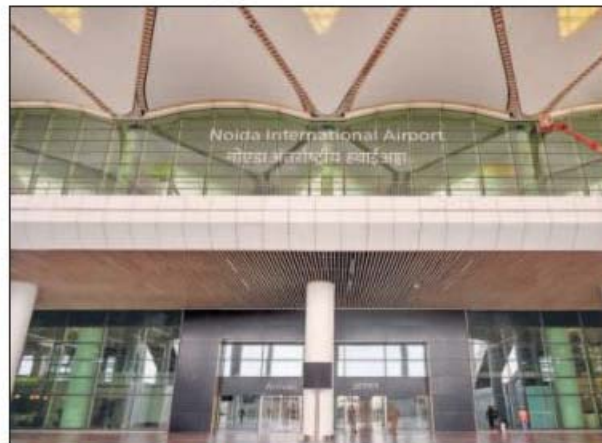
The start of services follows the approval for the Aerodrome Security Programme earlier this week.
