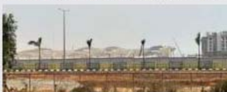
LAST STRETCH. The main terminal of the airport, which is nearing completion. A 6-km highway link is also under construction. (G NAGA SRIDHAR)
