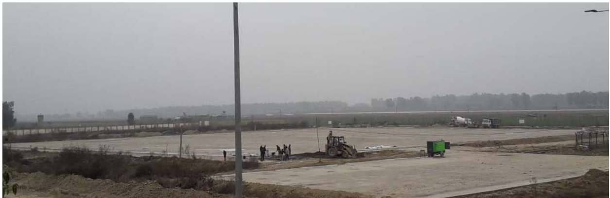
c) Top View of Apron and Ground Support Equipment Area (GSE)
