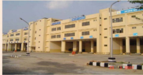
(Citiside view of Cargo Terminal, Kolkata Airport)
